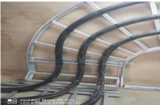
Substation Cable Racking Network
