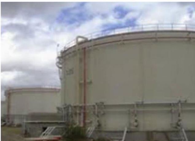
Tank Erection & Maintenance
