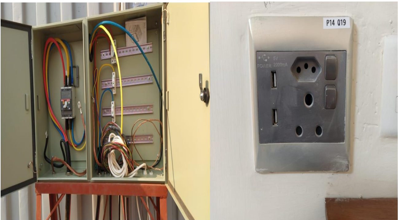
MetalKol Inkwazi Management Camp Distribution Board construction in progress
