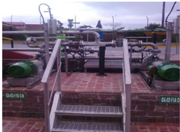
Pump, stairs & handrail installation
